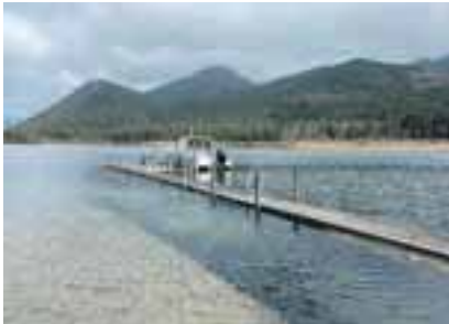
The jetty at Lake Rotoroa. Note how high the lake is and the concrete boat ramp under water.
